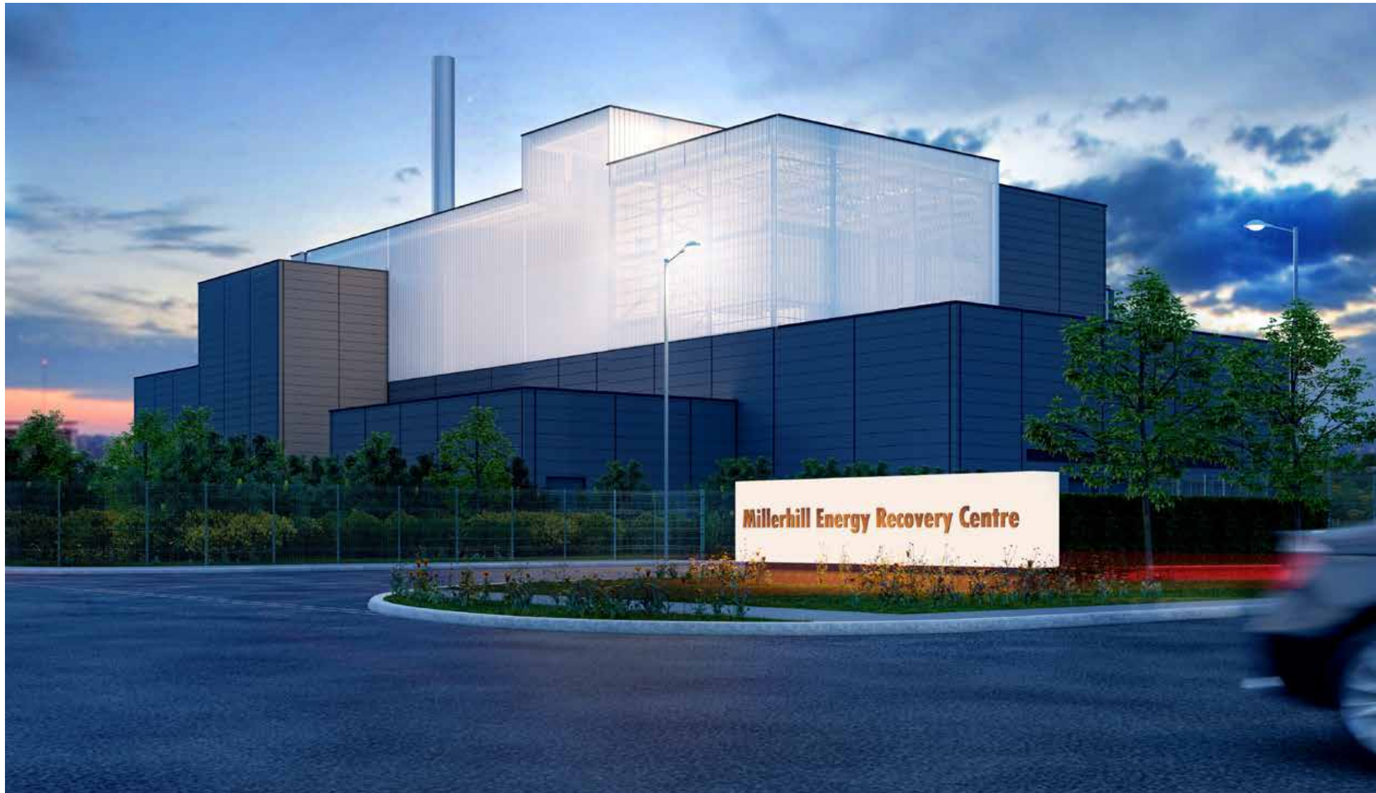
Millerhill Energy Recovery Centre Scotland, UK
